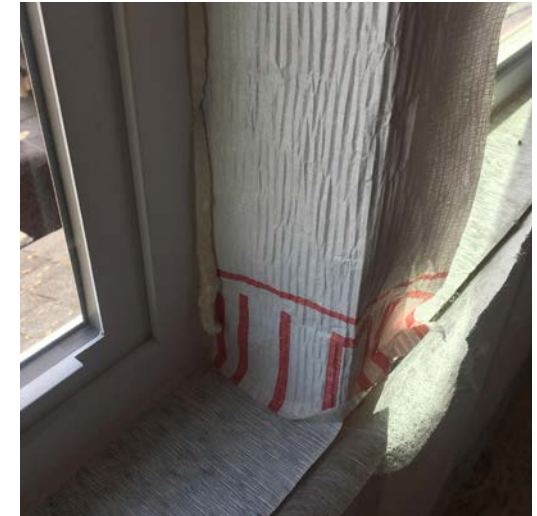
^ Foam sealing around window framing
